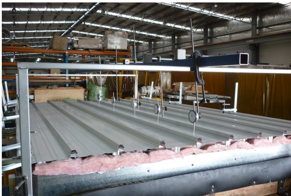
Figure 3. Installed sheet prior to serviceability testing.
