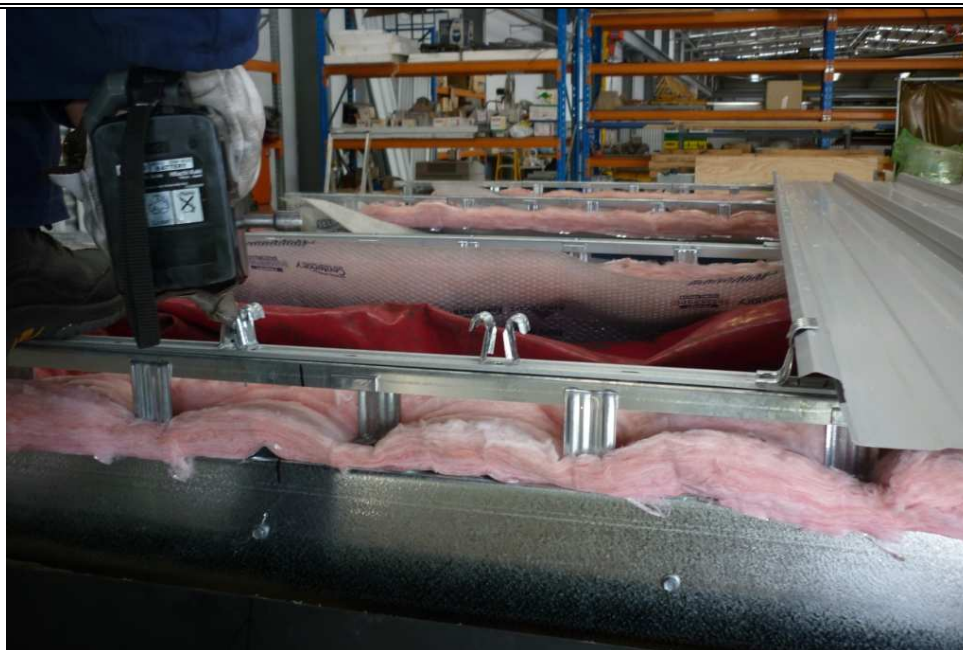
Figure 2. Installation of the sheet to spacers.
